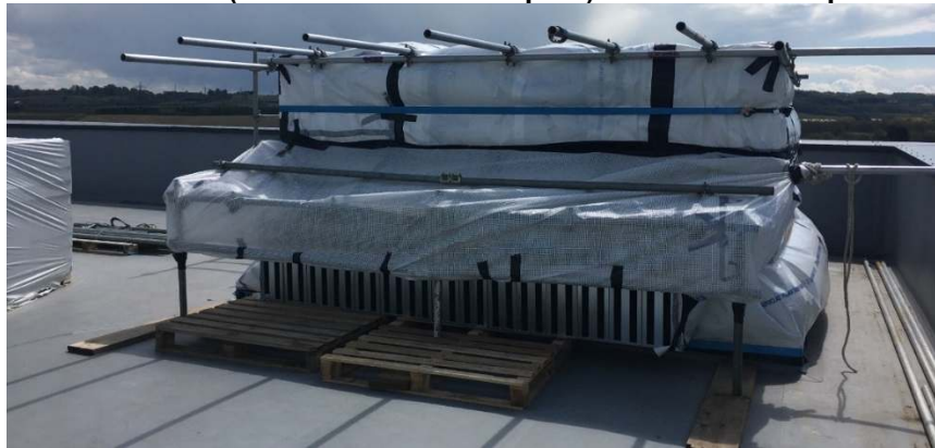
Photo 2: Temporary Sealed Canopy over a roof opening with scaffolding to secure shelter during high winds. Replacement filters (once filter media is spent) shown to left of photo
